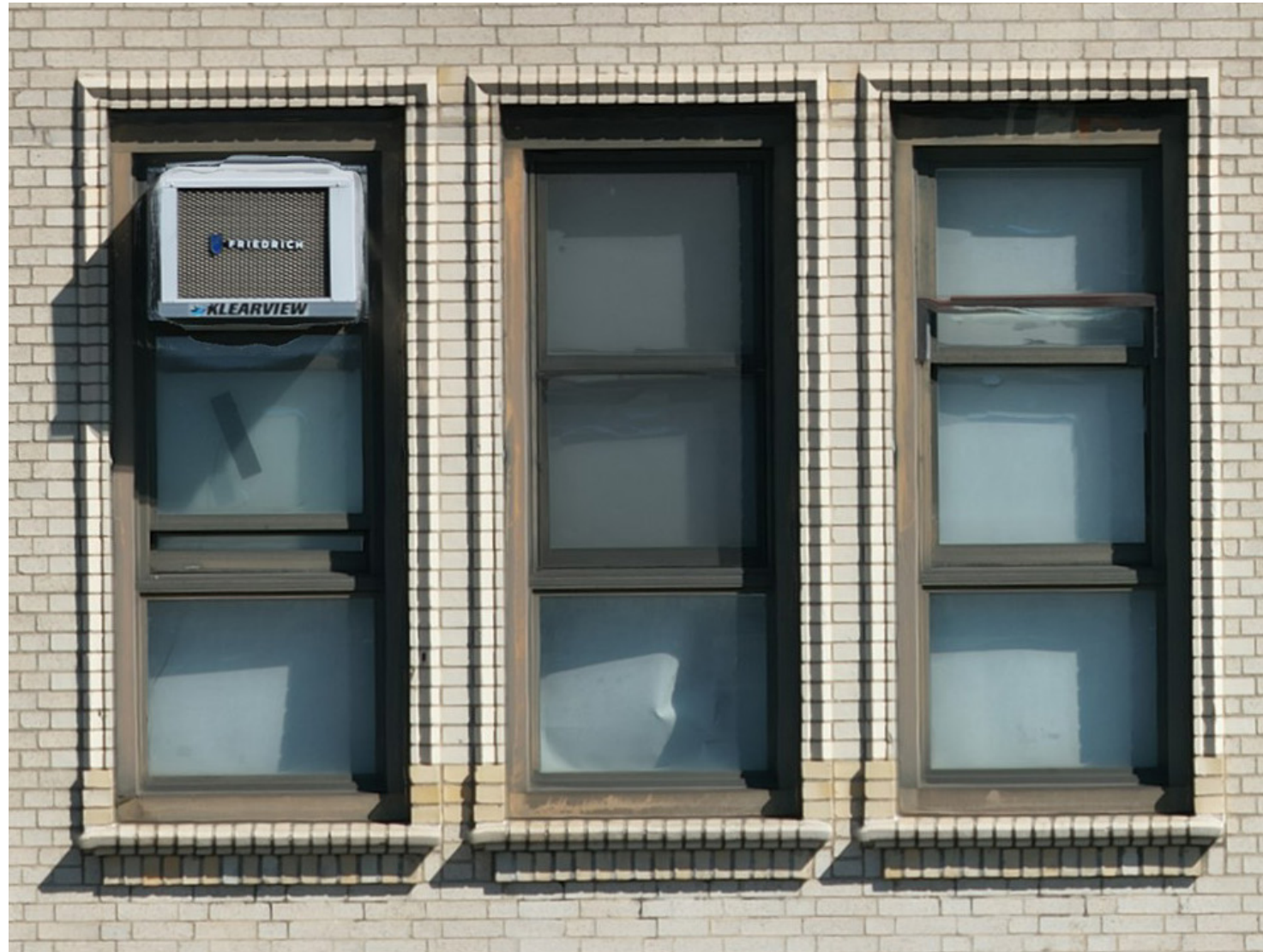
Typical Existing Windows at Street Facades
