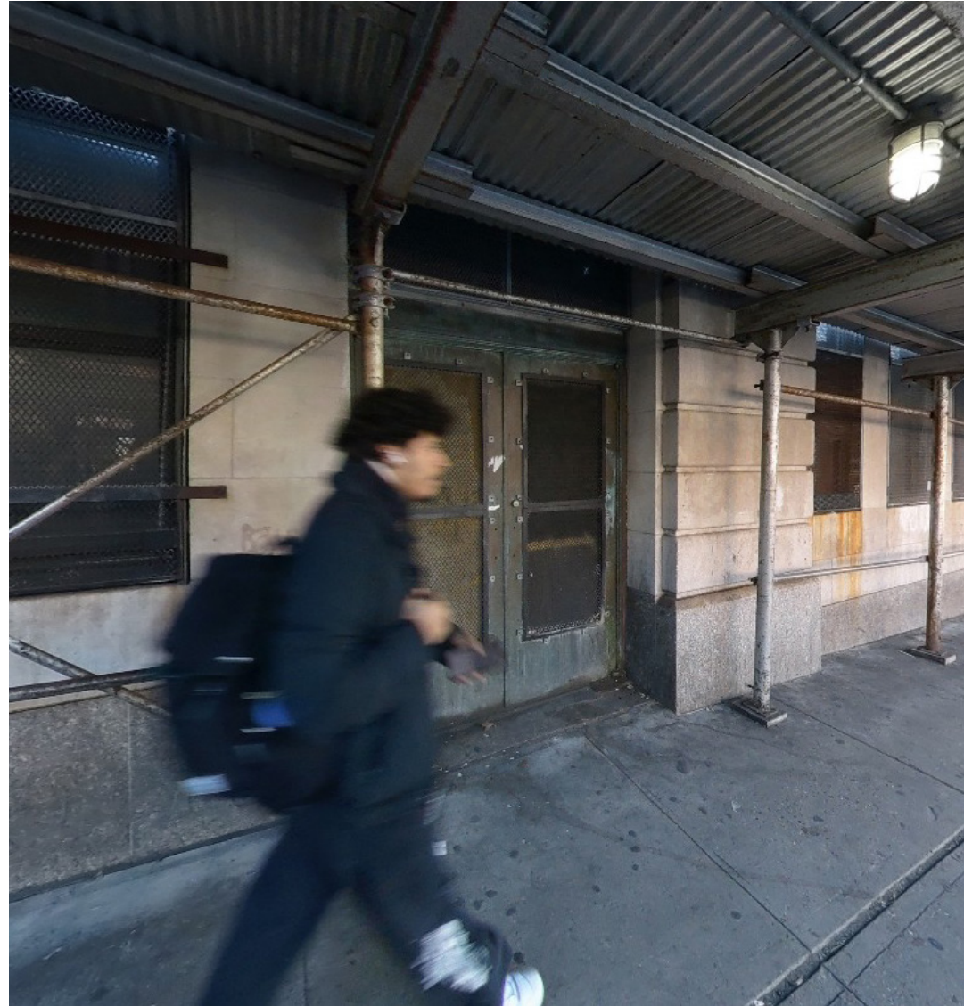
16: Entrance Door on E. Tremont Ave
