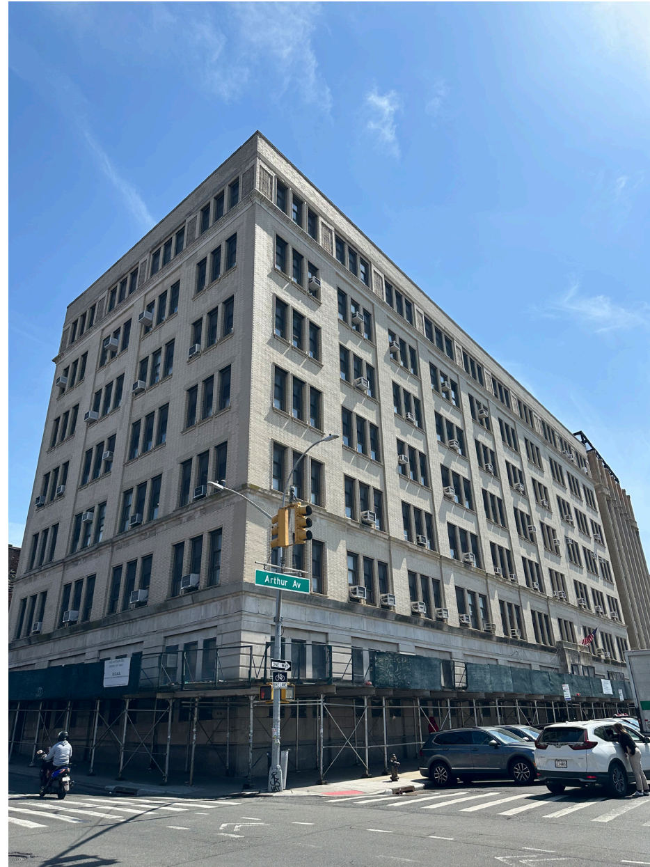
1: Northwest Building Corner at E. Tremont Ave and Arthur Ave
