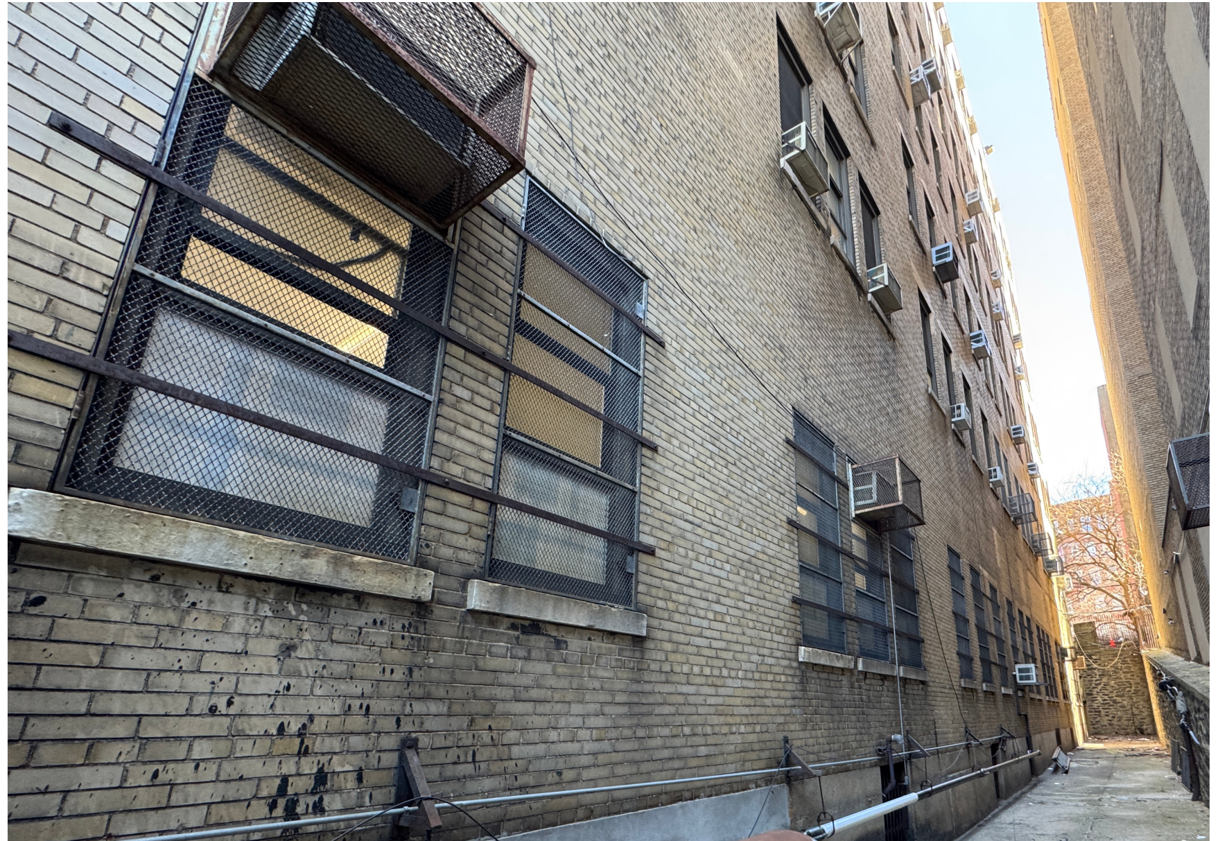
8: View of South Elevation at Rear Yard
