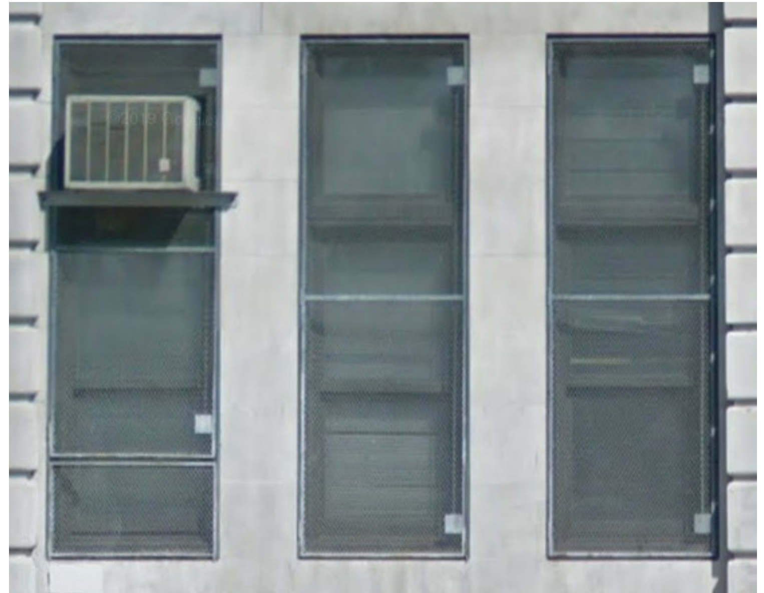
Typical Existing Window Grille at Street Facades
