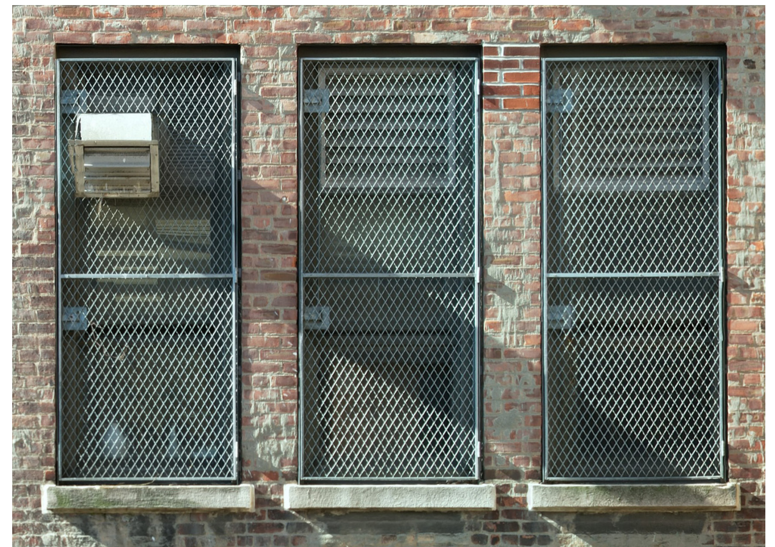
Typical Existing Window Grille at Rear Yard Facades
