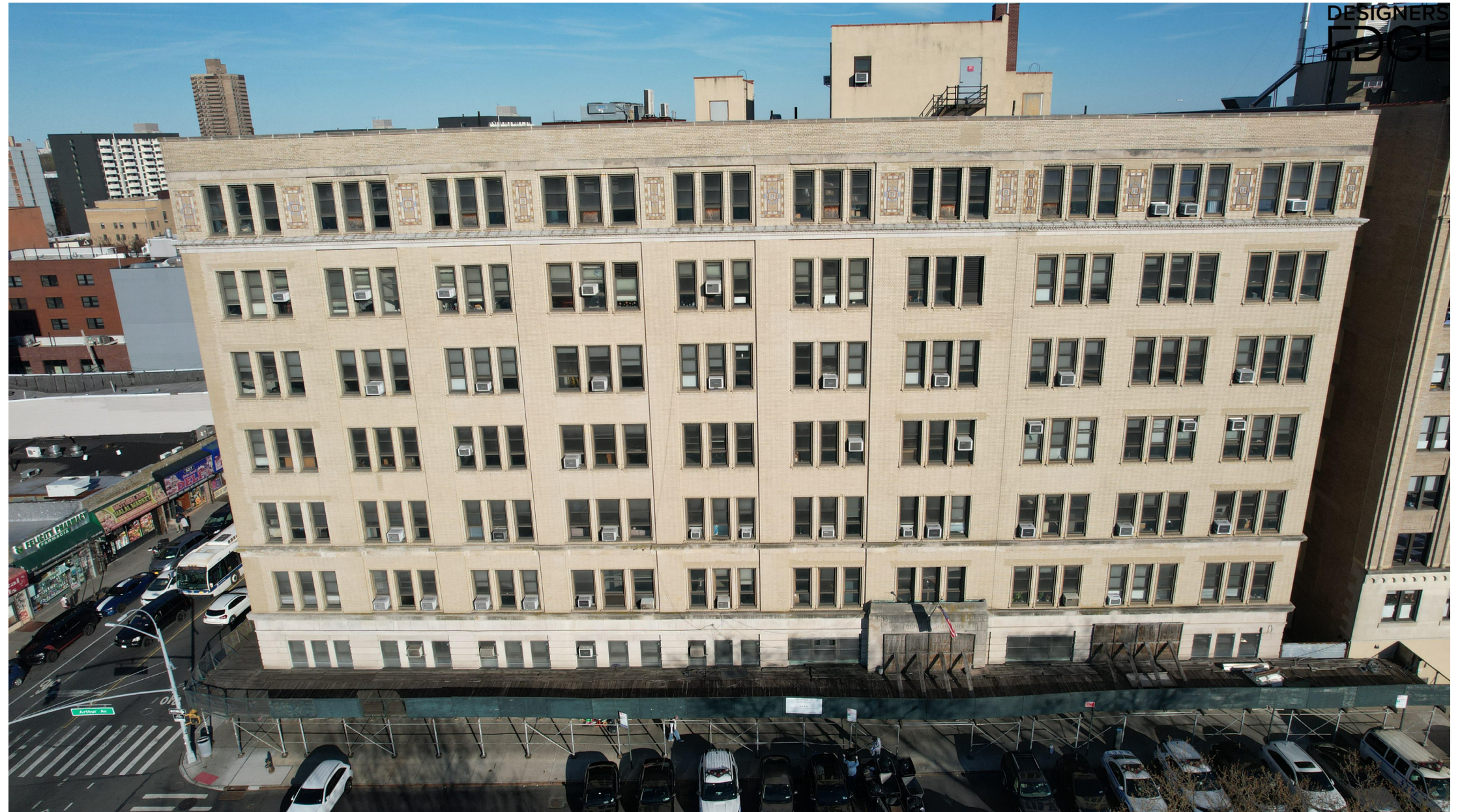
3: View of West Elevation at Arthur Ave
