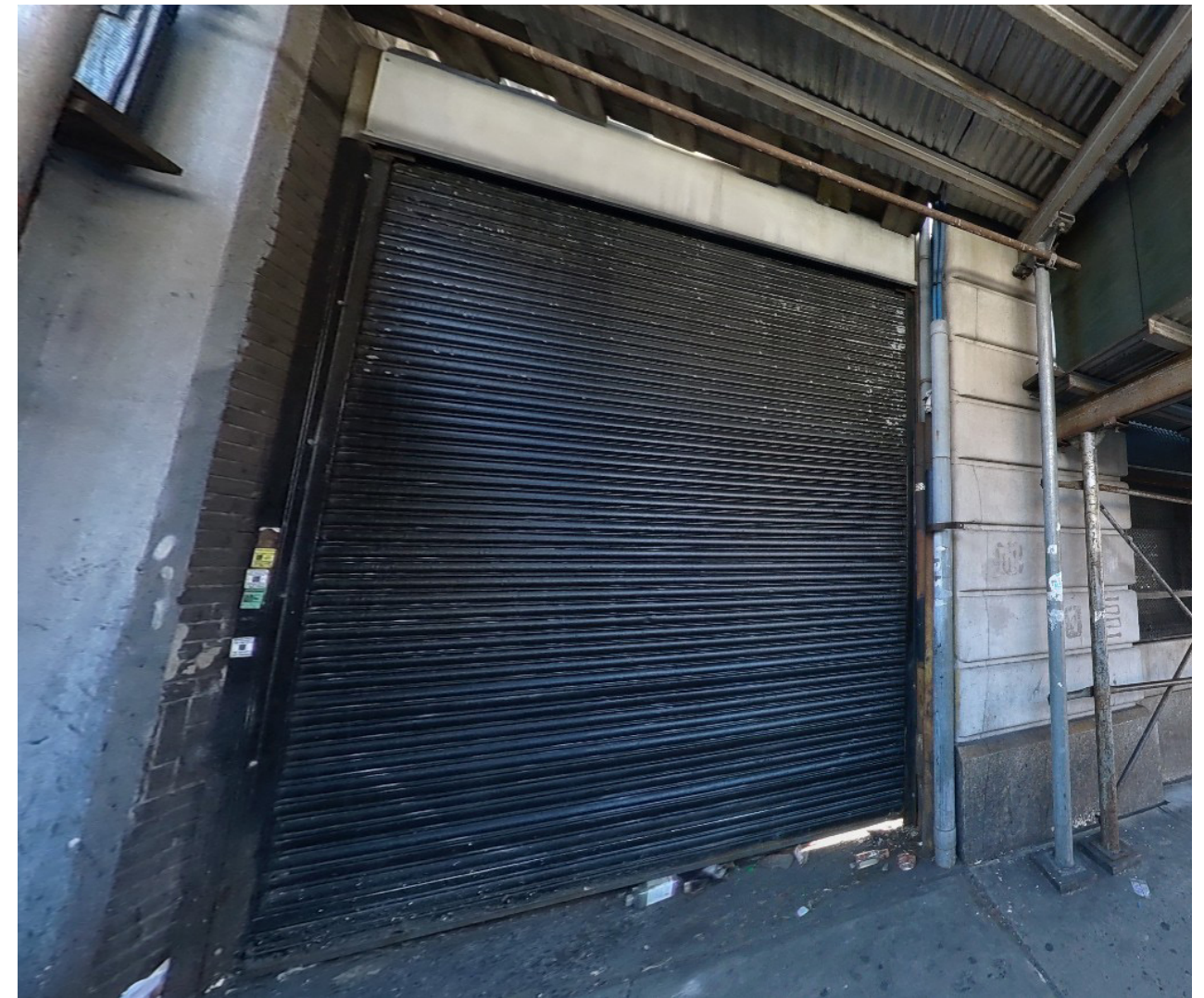
18: Roll-up Security Door on E. Tremont Ave
