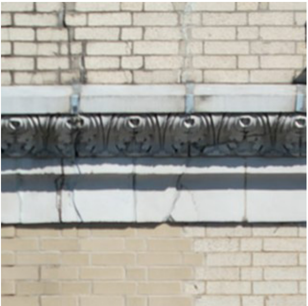
Terra Cotta at Street Facade
