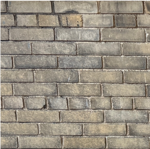
Common Brick behind Rainscreen Facade
