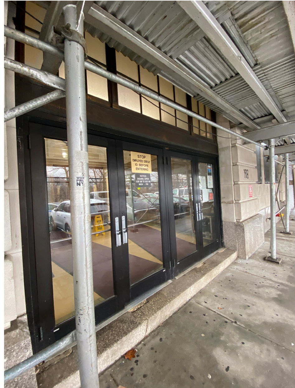
15: Entrance Door on Arthur Ave no. 1918
