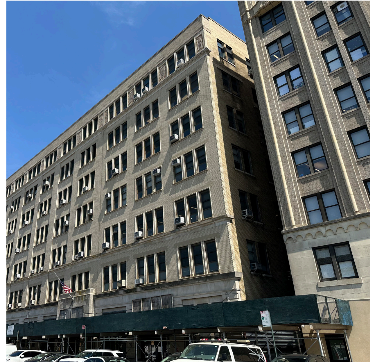
2: Southwest Building Corner at Adjacent Building on Arthur Ave
