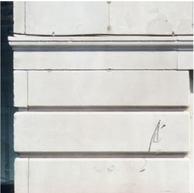
Limestone at Street Facade
