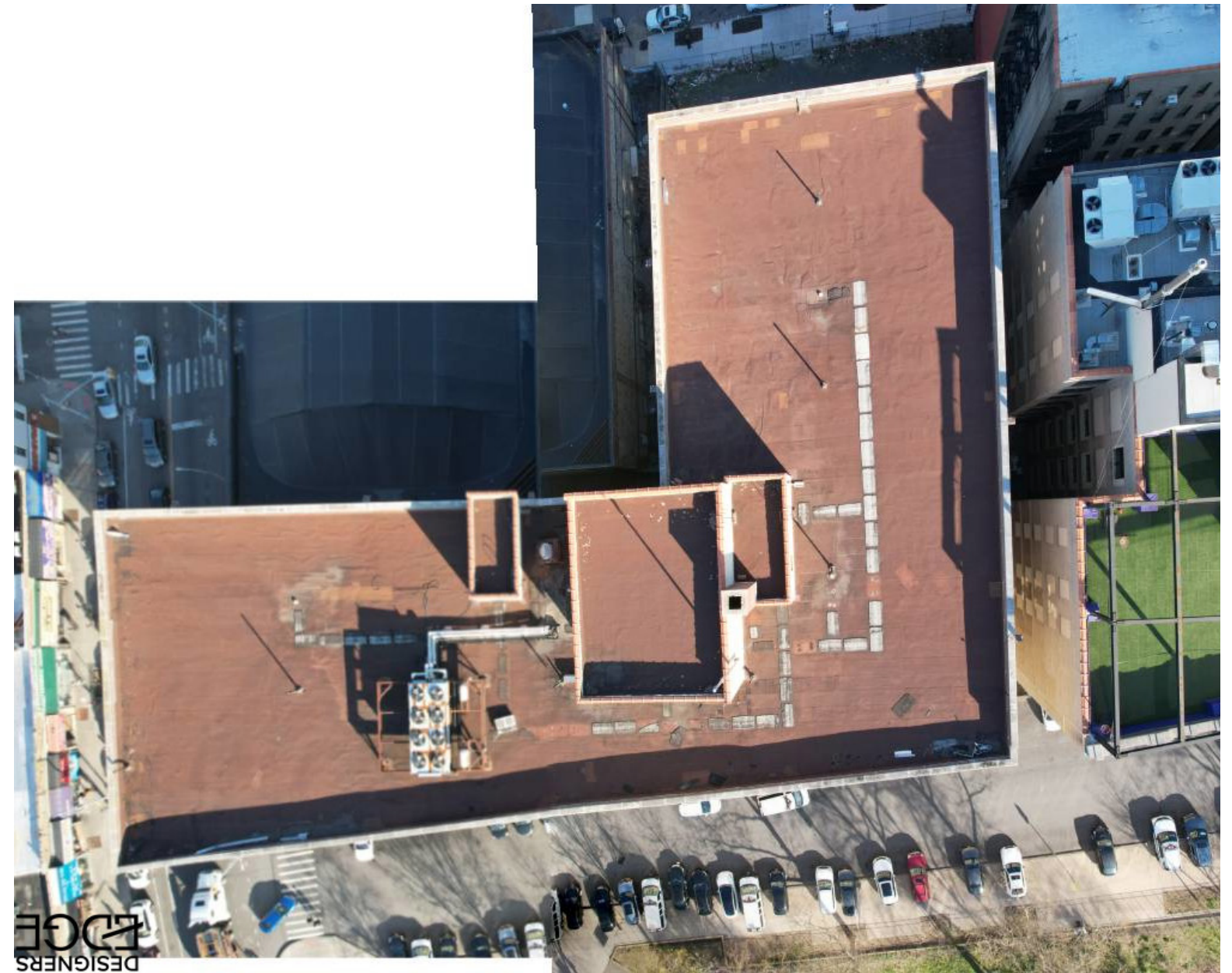
9: Aerial View of Roof
