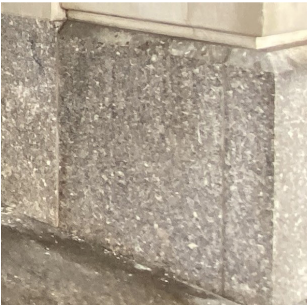
Granite at Street Facade
