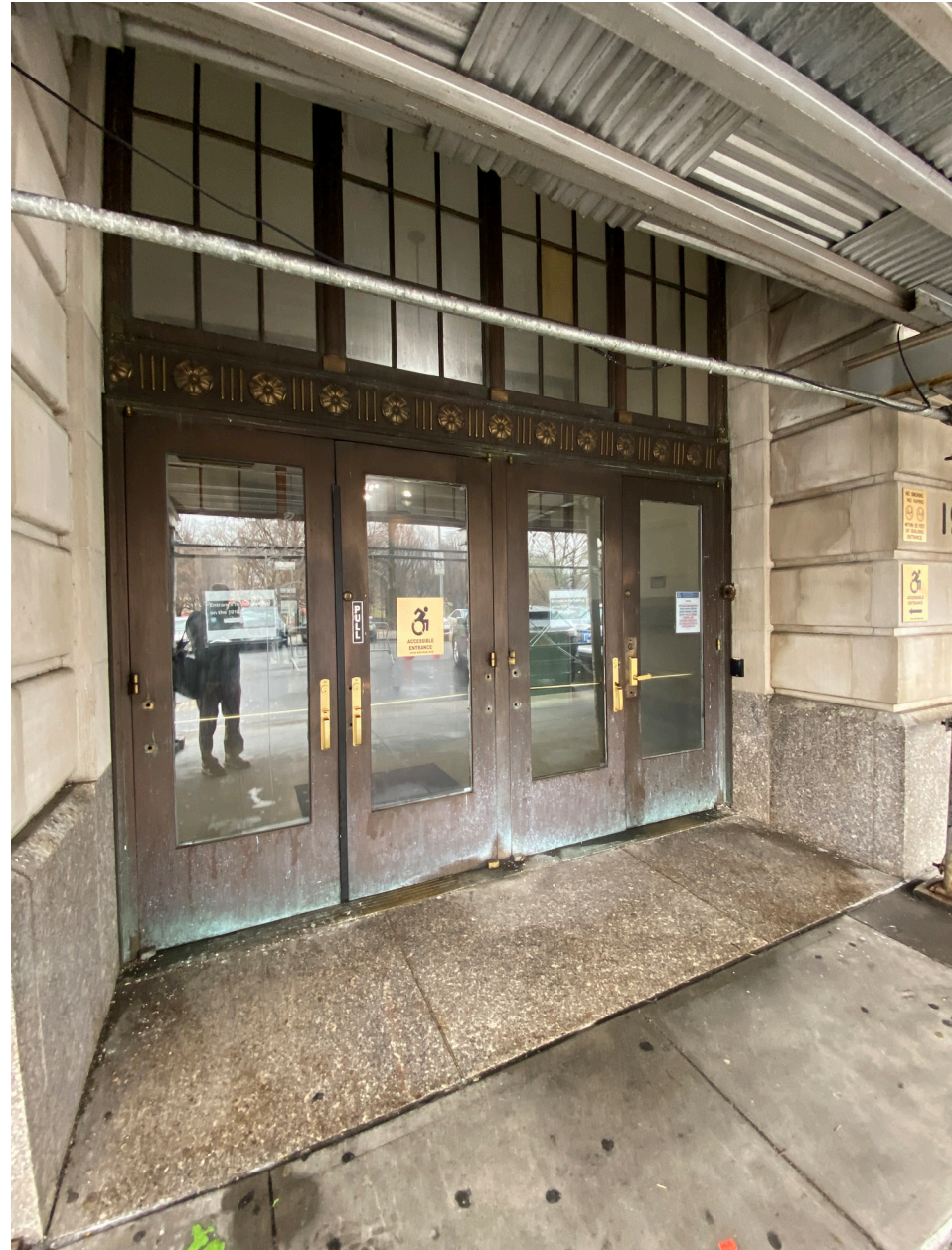
14: Entrance Door on Arthur Ave no. 1932
