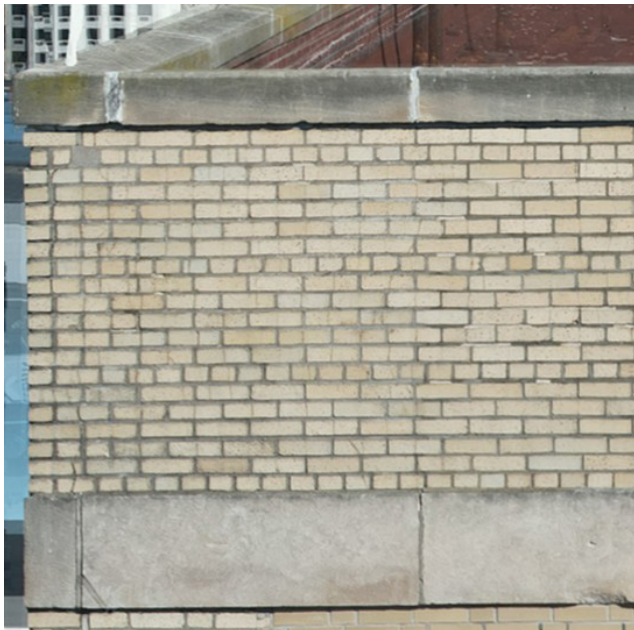
Concrete at Street Facade
