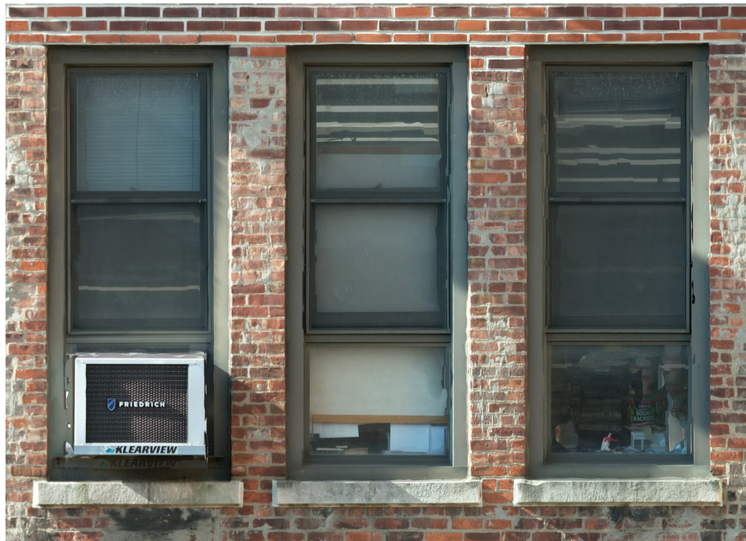
Typical Existing Windows at Rear Yard Facades
